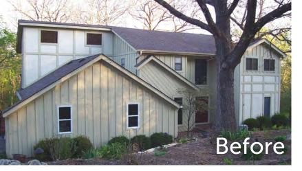
need for visual consistency as one approached the home. As a result, the garage façade also received new horizontal siding and a new window. The front facade had an oversized wall on each side with the roofline jutting out an additional 4 ft. to cover the sections of wall. This created 6 by 6 ft. of wasted space near the front door that blocked natural light into the home and an odd exterior treatment at one corner of the garage. The protruding wall was cut down to the foundation, and the
